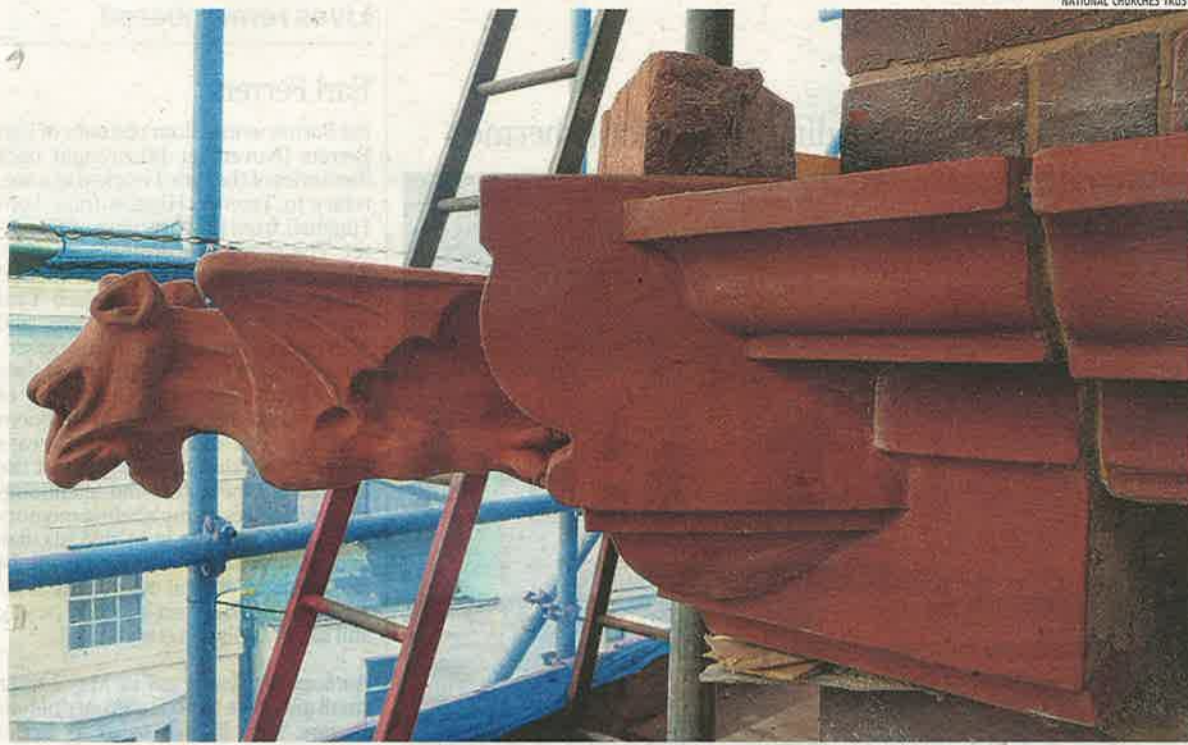
The skilful reproduction of terracotta on the Chapel Royal in Brighton earned HMDW Architects the Gold Medal, below
